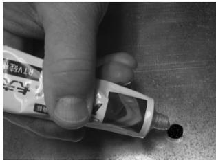
Apply a generous amount of silicone around holes before mounting adapter bases
